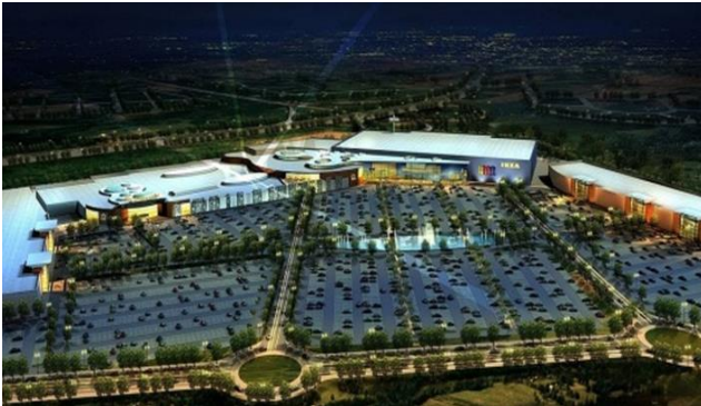
CENTRO COMERCIAL RIO SHOPPING VALLADOLID
